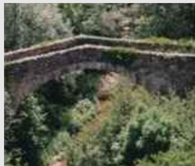
Vallfogona Medieval Bridge.
